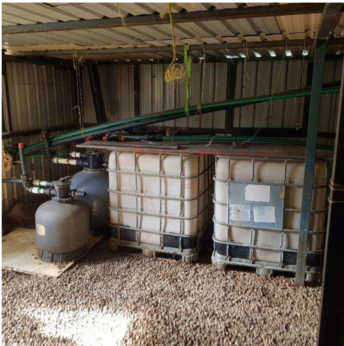
Figure 12: Hatchery Shed- Filtration Plant room (not installed) for recirculating system to hold harvested fingerlings and hold yabbies.
